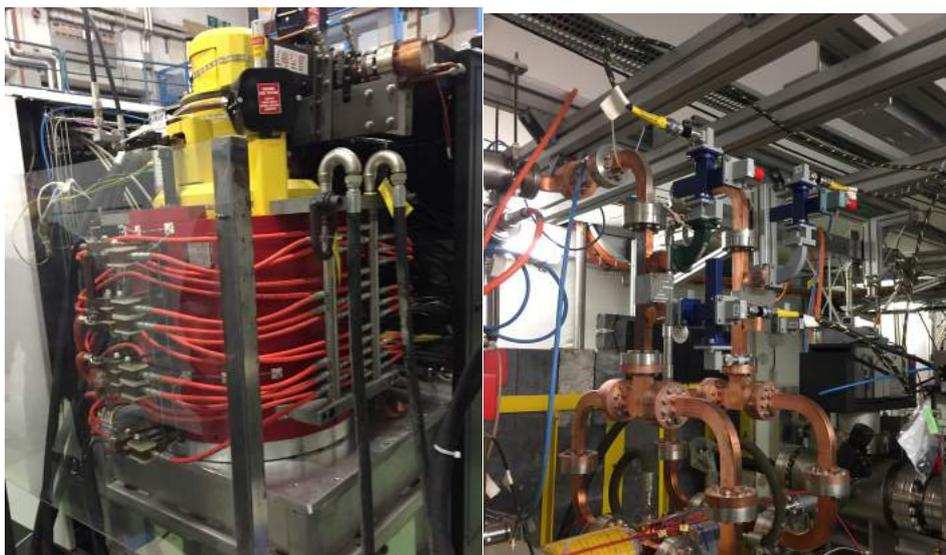
Figure 8: The klystrons of the CERN X-band facility.
