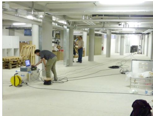
Figure 16: Basement of the new guest house with pylons (point 3).
