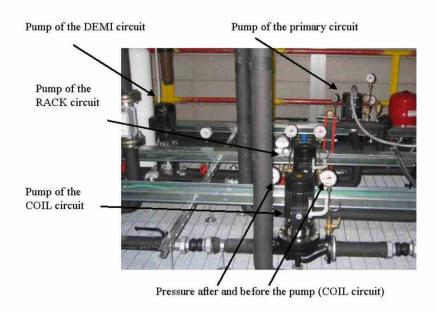
Figure 8: The pump system on the top platform.
