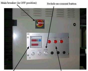
Phase current and voltage monitor R,S,T phase presence lamps
