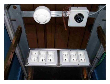
Figure 6: Temperature and smoke sensors. The knob allows the regulation of the overtemperature alarm threshold. The back of the distribution box and the corresponding plugs are also visible.
