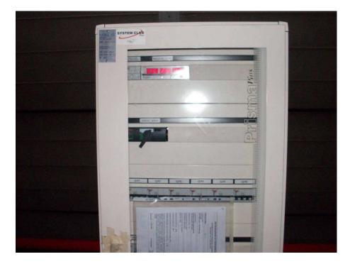
Figure 3: The main power switch.
