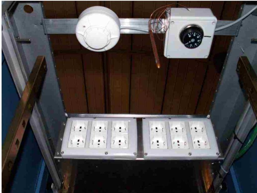
Figure 6: Temperature and smoke sensors. The knob allows the regulation of the overtemperature alarm threshold. The back of the distribution box and the corresponding plugs are also visible.
