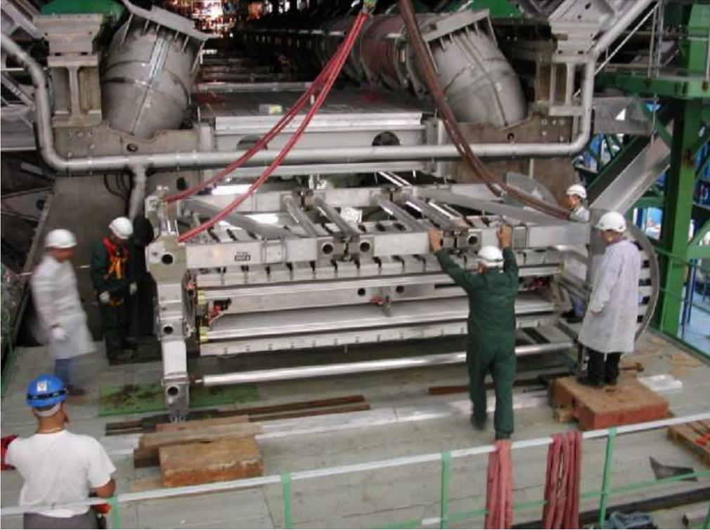
Figure 4: *The sliding of a BML station in the Atlas apparatus.*
