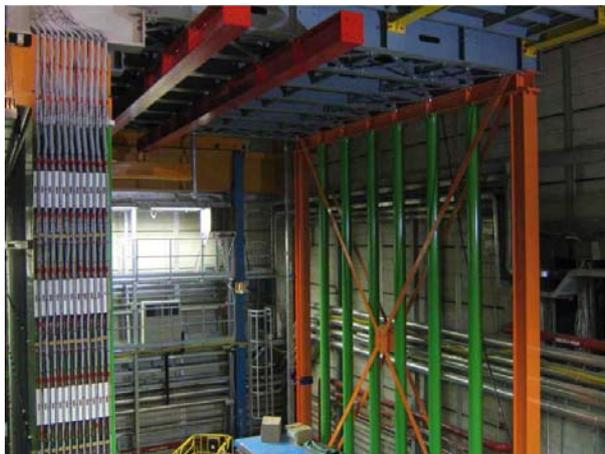
Figure 2: Seismic support structure at the back of OPERA.
