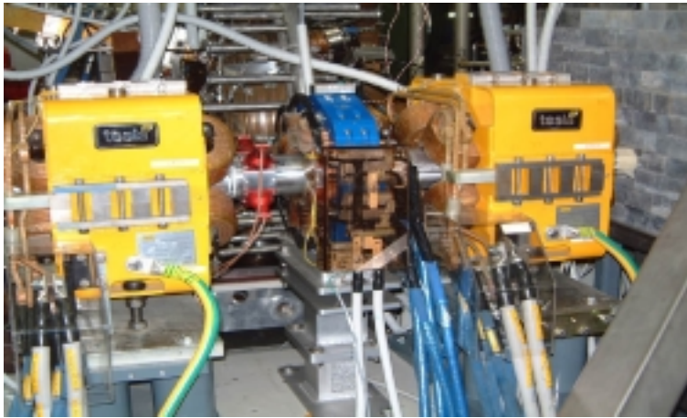
Figure 2: Octupole magnet (blue) installed in DAΦNE.
