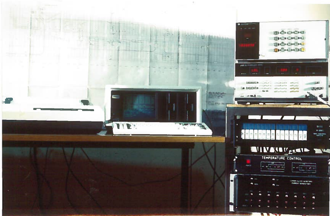
Fig.5 - Photograph of the control system
