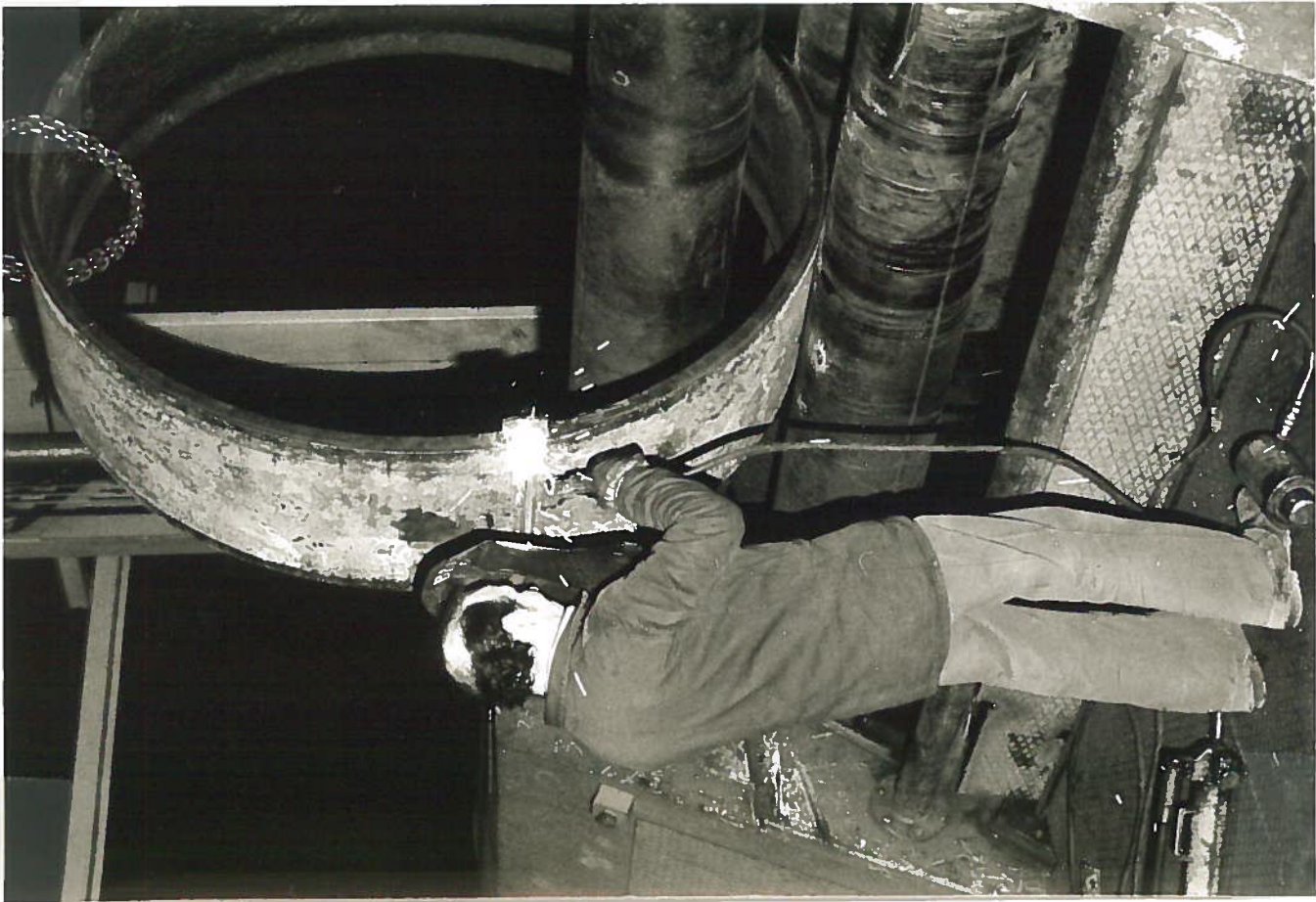
FIG. 61 - View of the ring during welding.
