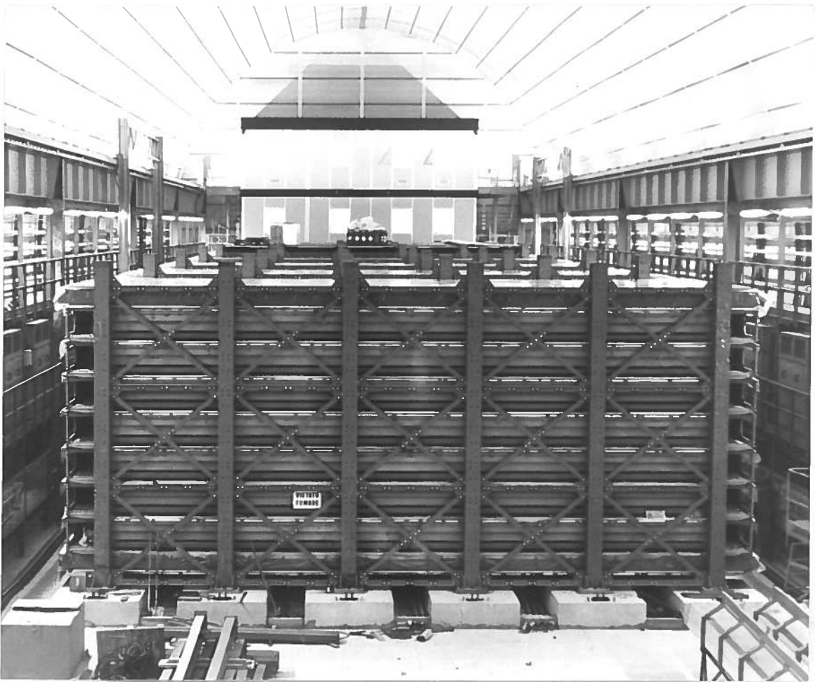
FIG. 3 - Photographic view of the first three supermodules of MACRO (total length 38 m). The first of these supermodules was used in the data reported here.
