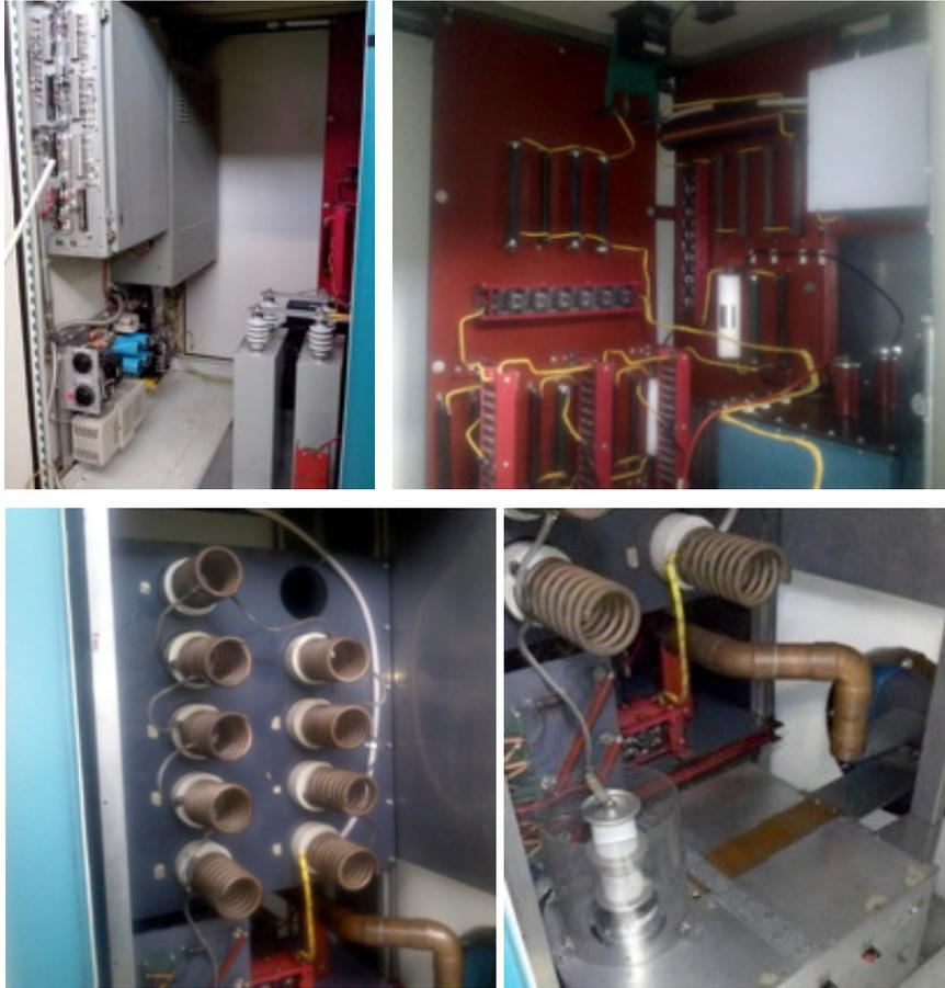
**Figure 3.3:** The SCR rectifier, the core bias and filament power supplies are placed inside one door of the modulator racks (top left), together with the diode arrays, the large charge capacitor and filters of the charging circuit (top right). In the other rack door: the 9 LC cells PFN (bottom left), the Hydrogen gas thyatron and the conductor towards the pulse transformer (bottom right).
