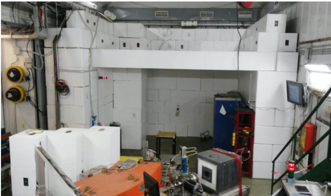
**Figure 2.10:** During the July-September 2015 shutdown the concrete block shielding of the BTF experimental hall has been dismantled and reinstalled in an improved configuration, adding a concrete ceiling (50 cm concrete).
