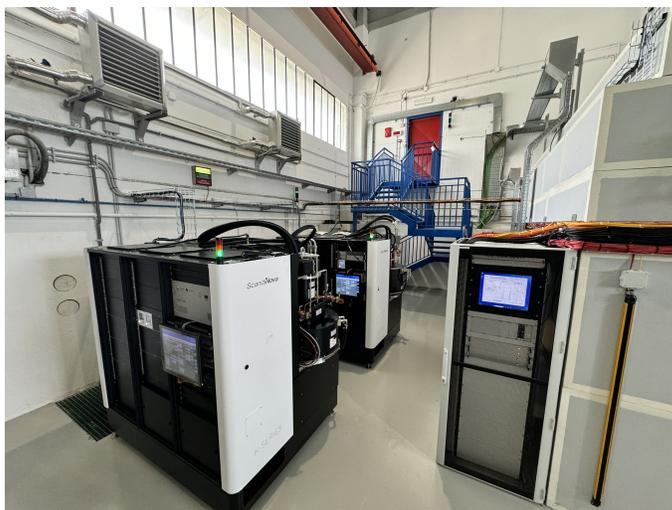
Figure 4: X-band and C-band high repetition rate RF sources installed at the TEX facility.
