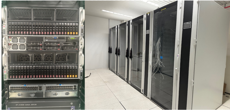
Figure 2: (Left) The two GPU-server (each equipped with three GPU NVIDIA Tensore Core A100 80 Gb) and one of the new switches (Right) The new white space and racks that will host the new STAR IT equipment.
