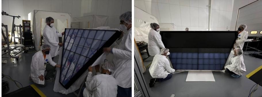
Figure 4: *The two sections of 2 cm thickness aerogel tile assembled on the frontal mirrors (left) and the 3 cm section assembled on the frontal closing panel (right).*
