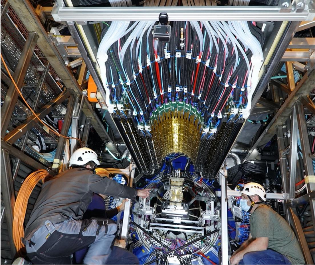
Figure 1: *Installation of the new Inner Tracking System in ALICE*
