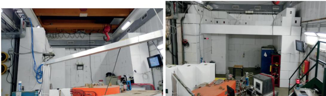
Figure 6: *Shielding blocks in the BTF experimental hall: before (left) and after (right) the re-arrangement and realization of the coverage.*
