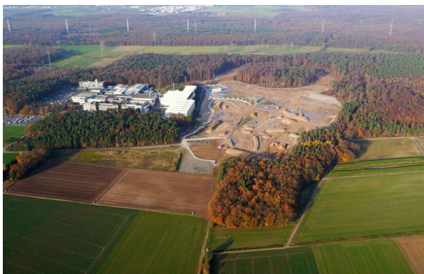
Figure 1: Aerial view of the FAIR construction site.
