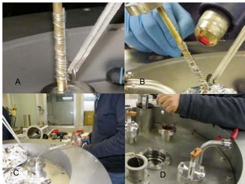
Figure 2: *Photographs taken during the soldering procedure of the superconducting cables and the installation of thermometers inside the cryostat.*
