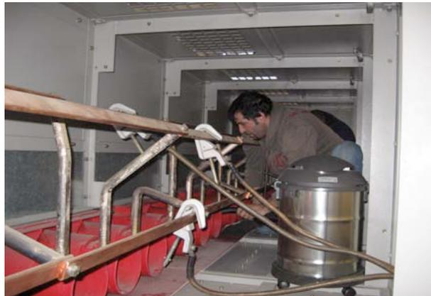
Figure 3: *MV switchboards internal maintenance.*
