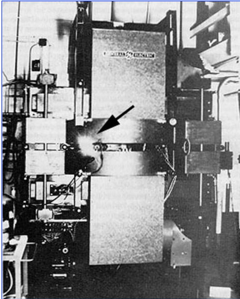
1947 General Electric Res. Lab. - 70 MeV Electron Synchrotron - N.Y. USA
