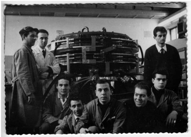
Fig.3 A few components of the AdA building team
