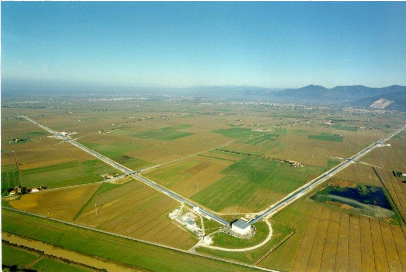
The effect of the GW is proportional to the length of the interferometer arms  $\rightarrow$  long arms are needed (3 km)
