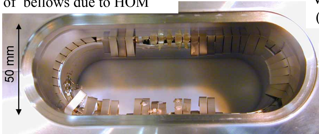
Damaged RF-shield fingers of bellows due to HOM
