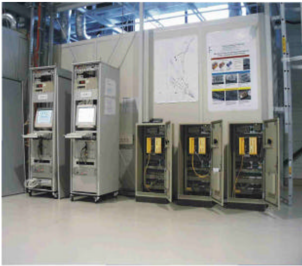
Figure3 right: three BPSS Cabinets for LIGA Beamlines
